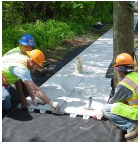
Laying out pavers prior to joining
