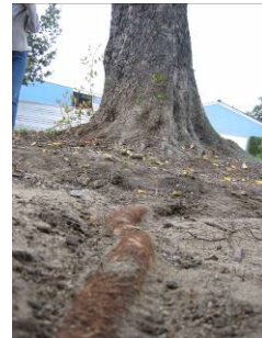
Directional root trimming, selecting roots safe to cut without endangering tree
