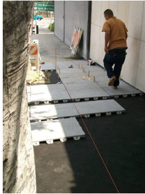
Laying out pavers prior to joining
