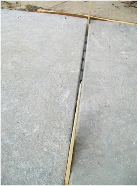
Pavers with wood shims to aid spacing
