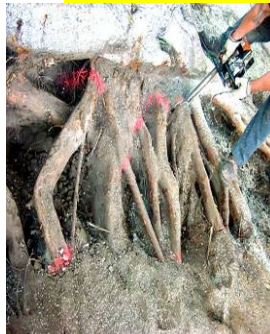
Directional root trimming, selecting roots safe to cut without endangering tree
