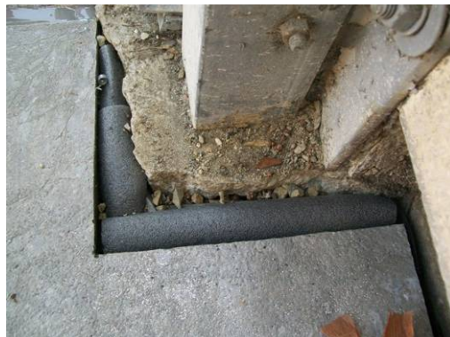
Foam filling for large seams
