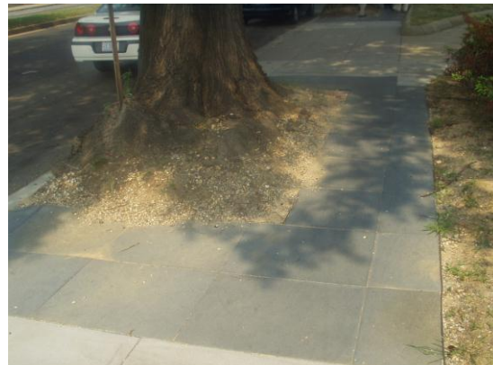
The left photo depicts the broken concrete sidewalks around the mature Oak trees on Rhode Island Avenue. The right photo depicts a Rubbersidewalks™ installation seven years later.
