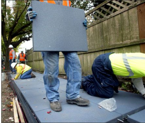
Rubbersidewalks installation
