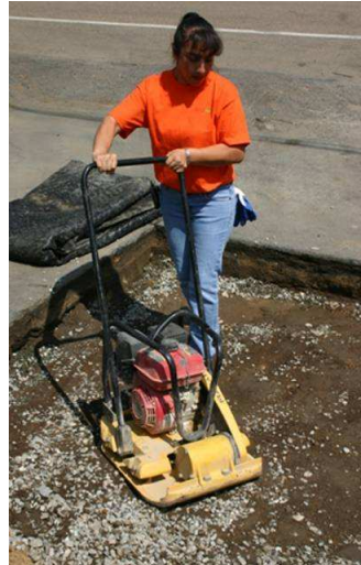
Class 2 permeable base illustrated
